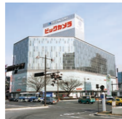
C Bic Camera The home appliances mass retailer is in a very convenient location in front of Okayama Station. It has three stories and a basement.
